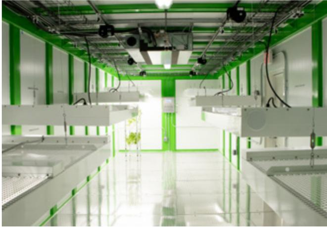
MineARC provided A&L Biologicals with a custom approach to air handling to reduce internal airspeed and improve air circulation in the unit without sacrificing fresh air exchange.
